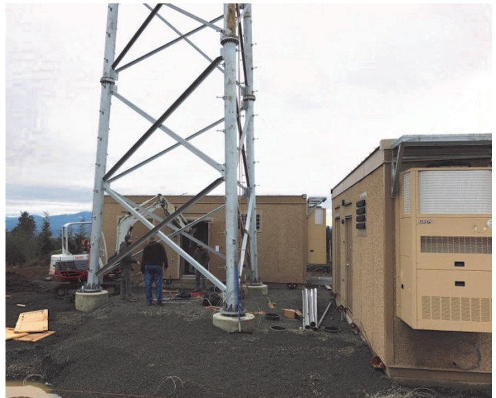
New "Reservoir" Site being constructed off of Pipeline Road.
